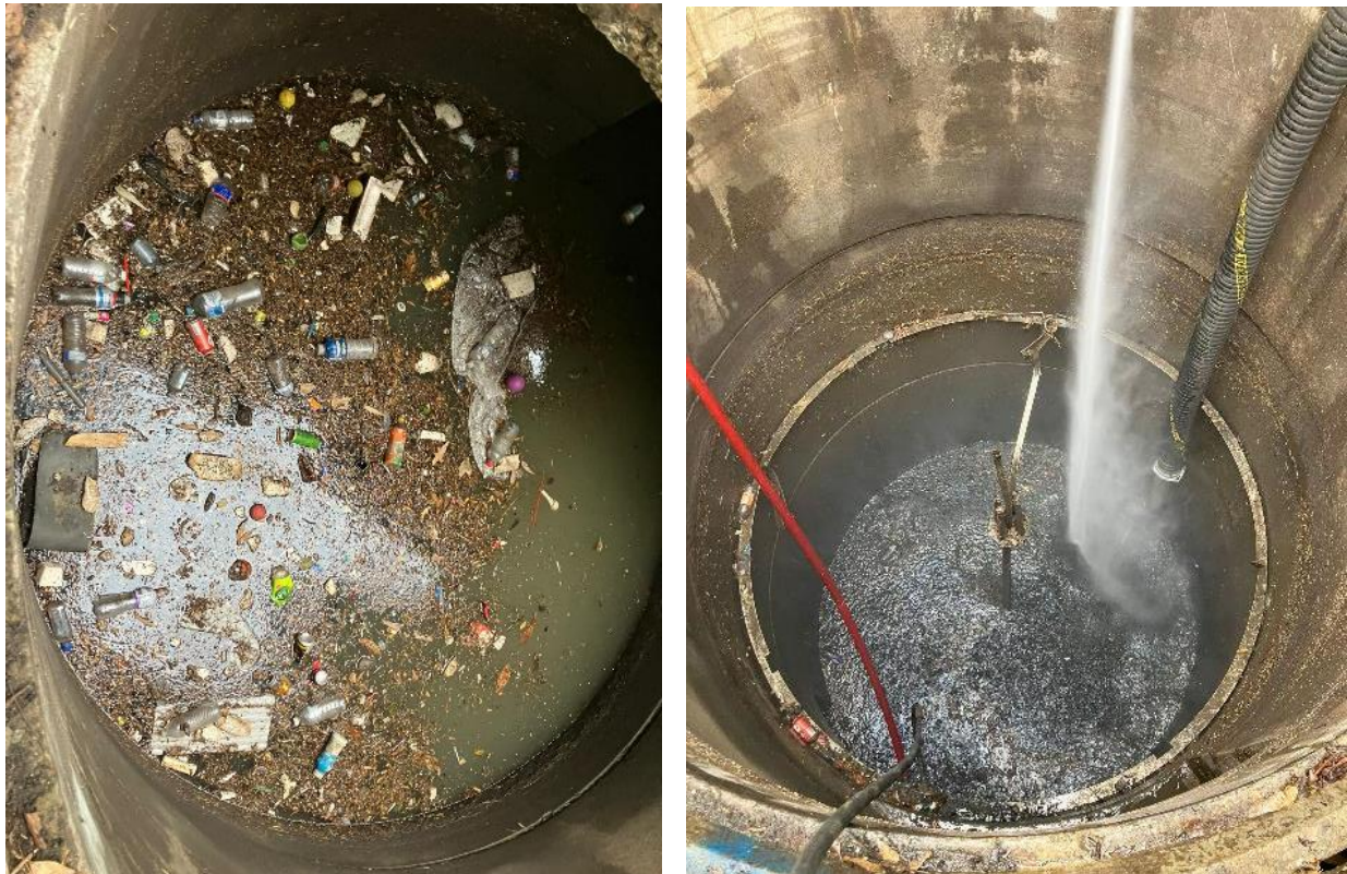
Photos of Gross Pollutant Trap (GPT) Canva Street Canley Vale (before and after clean)
